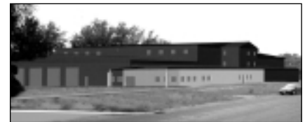
Proposed Saint Peter Wastewater Treatment Facility
