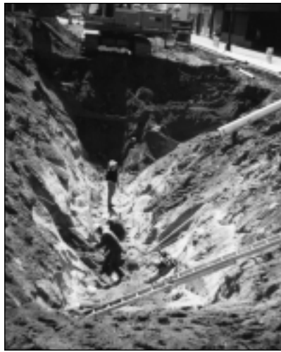
Sewer and water main replacement in New Ulm.
