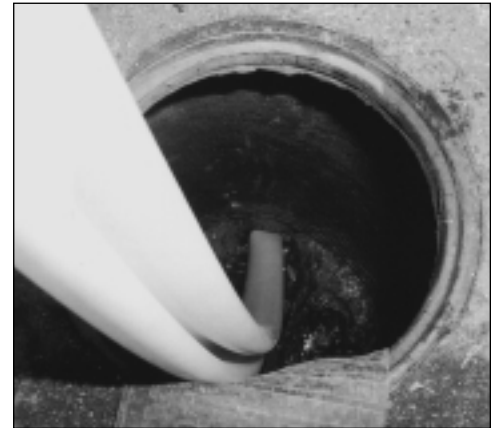
Pulled through the damaged pipe, the U-Liner is a safe & economical.
