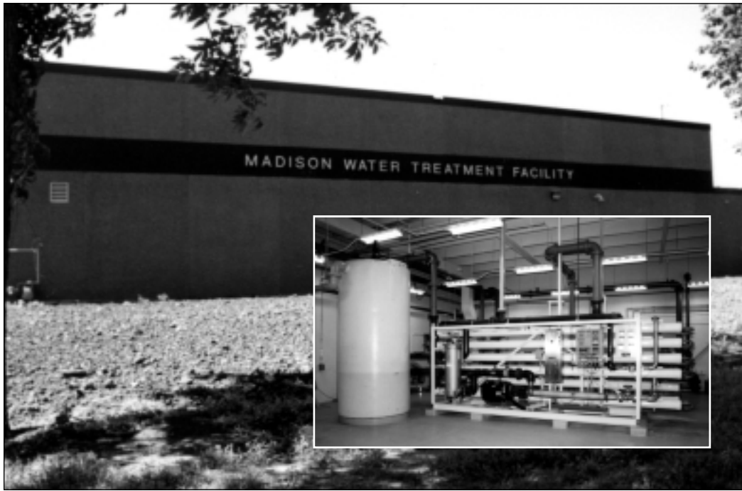
A new water treatment plant in Madison, Minnesota uses an innovative reverse osmosis system.
