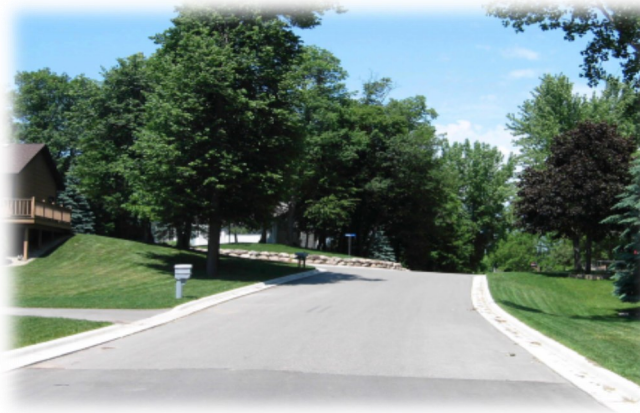
Brooksville Hills after reconstruction
