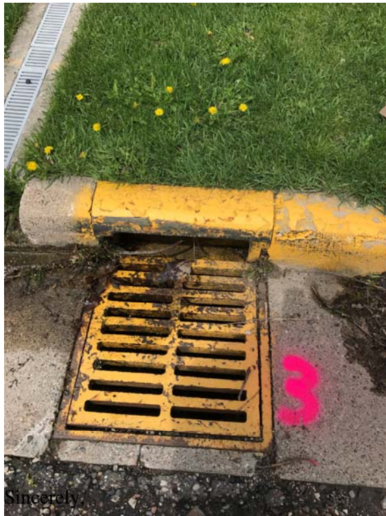
Catch Basin with Inadequate Grate Capacity
