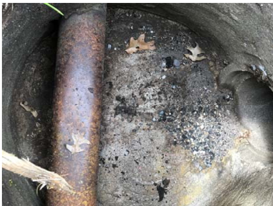
Catch Basin with Pipe Through it
