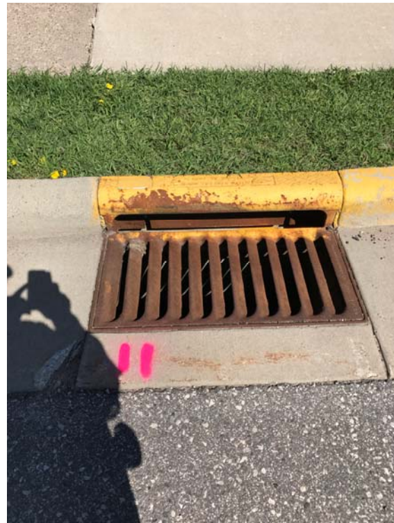
Catch Basin with Adequate Grate Capacity – Williams Street Project.
