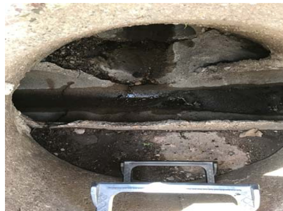
Catch Basin in Very Poor Condition
